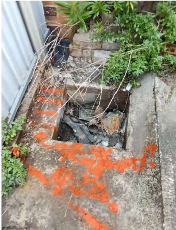
Photo 5: Drainage pit in north east of the site
